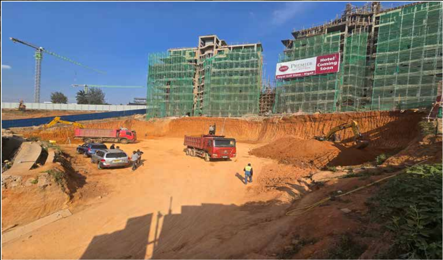
Block C Construction works in progress: July 2025
