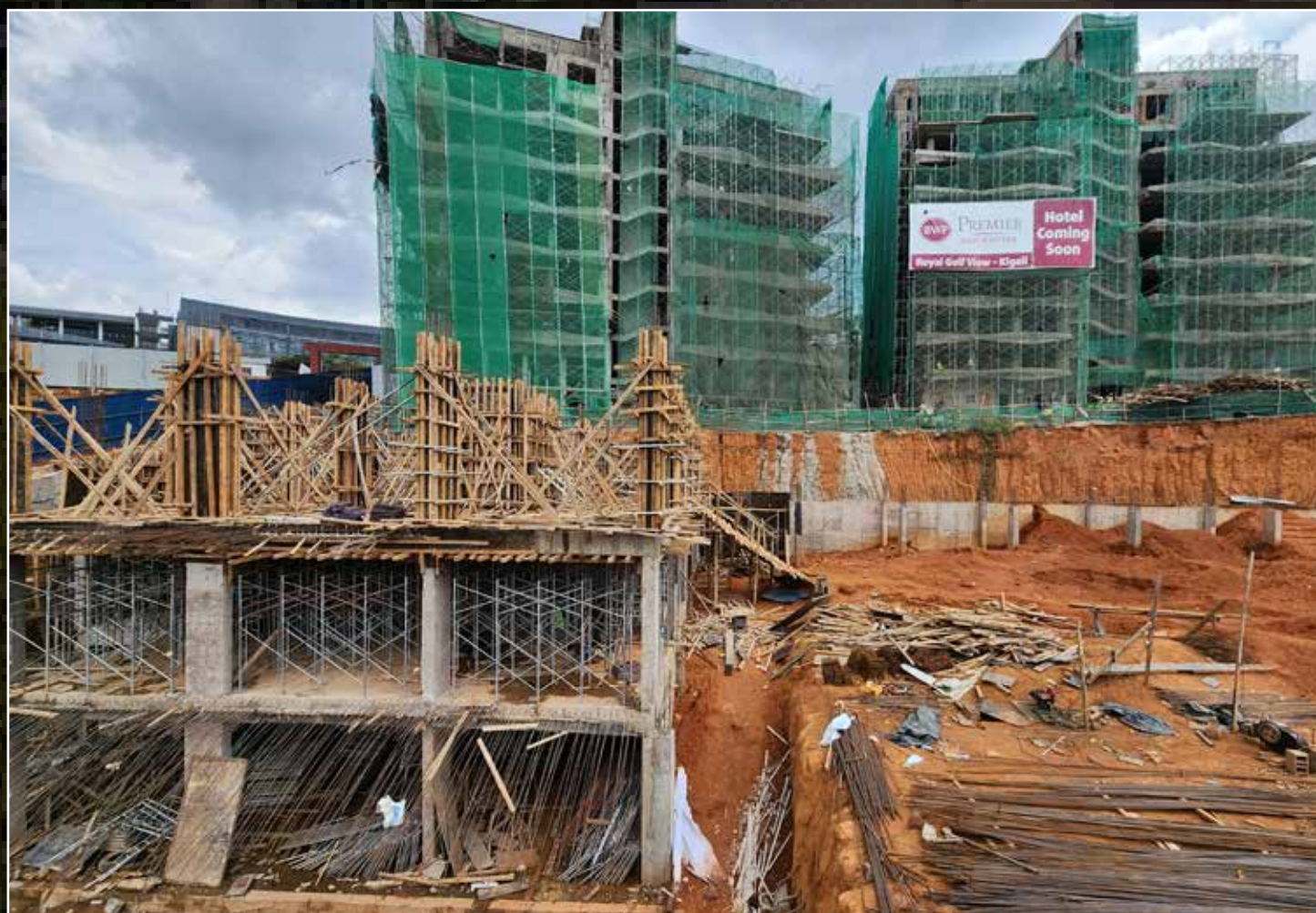
Construction for Block C (Hotel Building) in progress OCTOBER 2025
